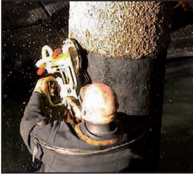
Cleaning with a power tool.
