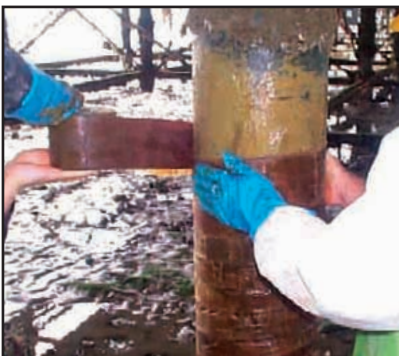
Applying Denso Marine Piling Tape.
