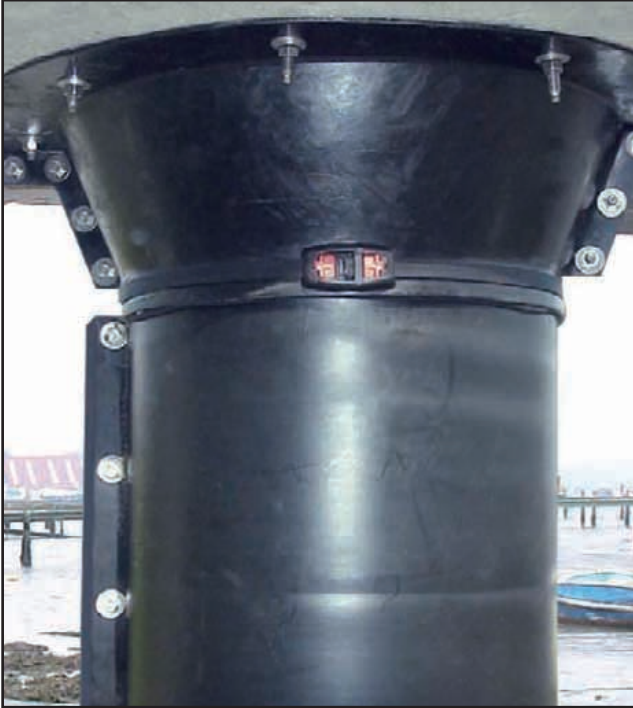
The Pile Cap is bolted to the underside of the jetty deck.
